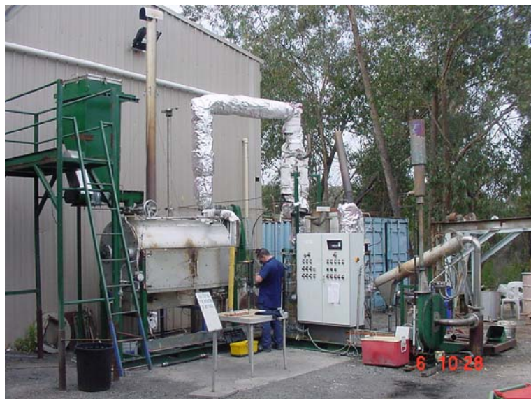
Figure 2. Photograph of the pilot plant.
